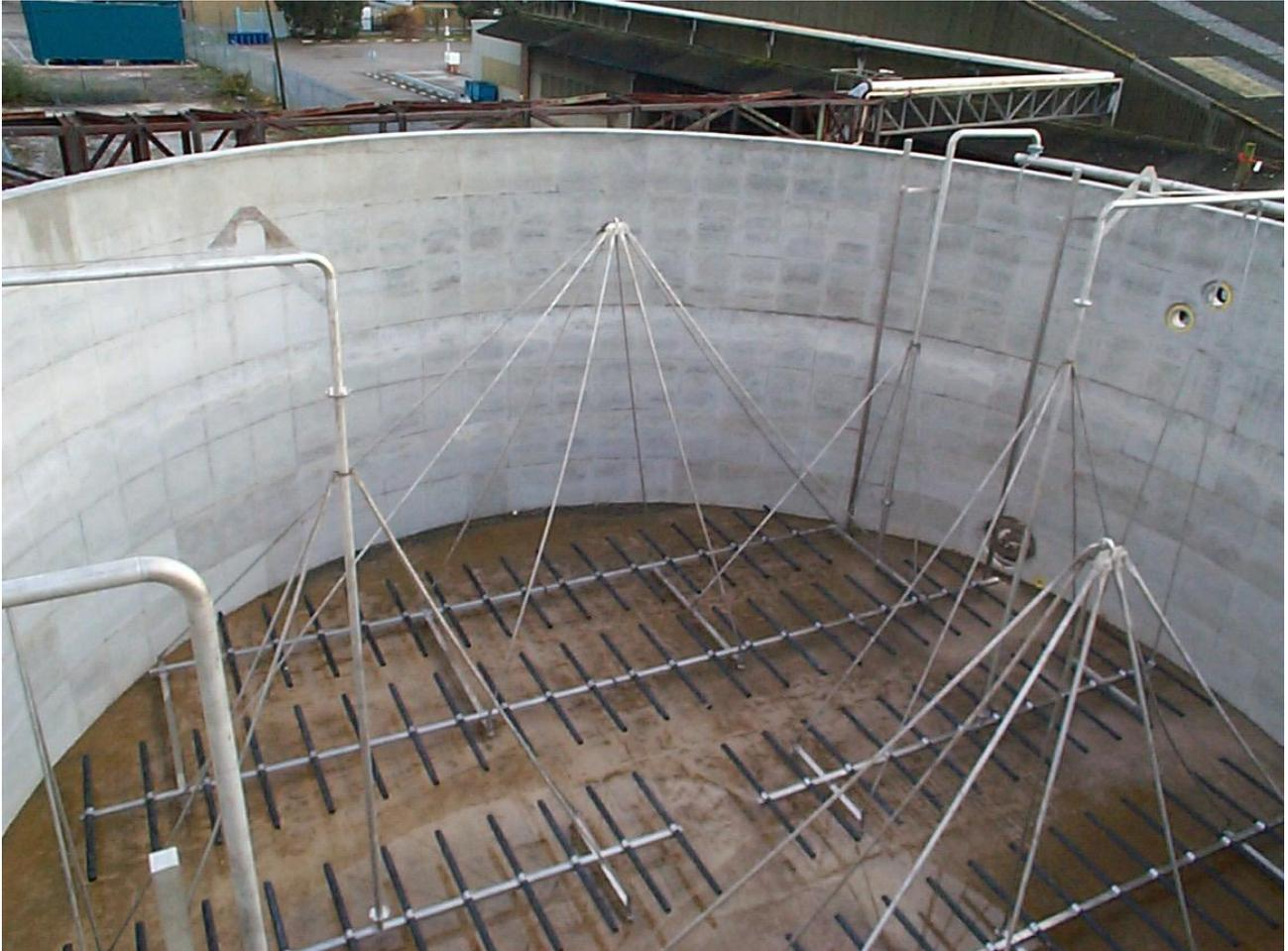
View of the removable tubular fine bubble aeration system within the Aeration tank
