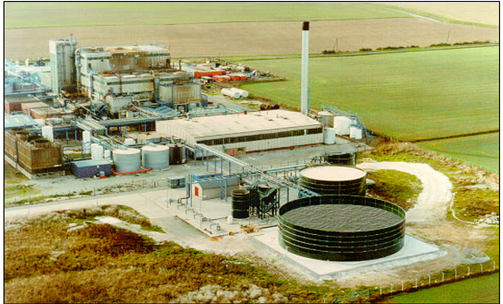
Aerial view of the treatment plant
