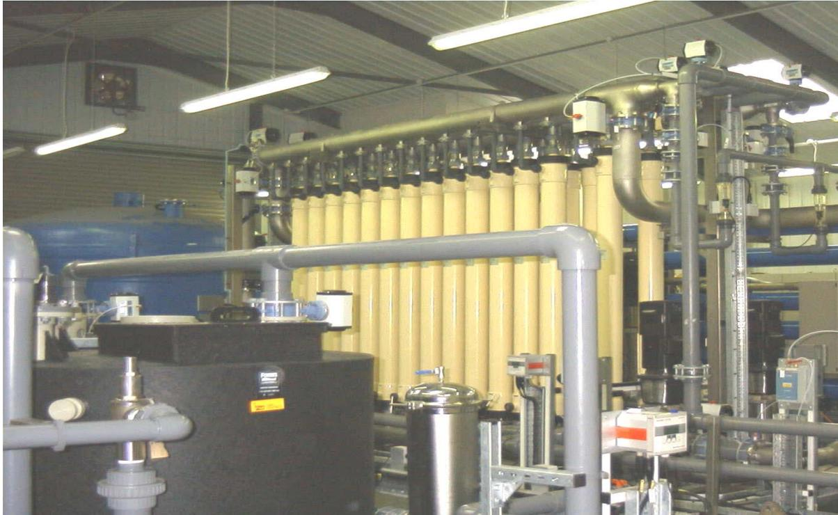
Twin stream microfiltration system, with Reverse Osmosis Plant in the background and CIP facility in foreground.
